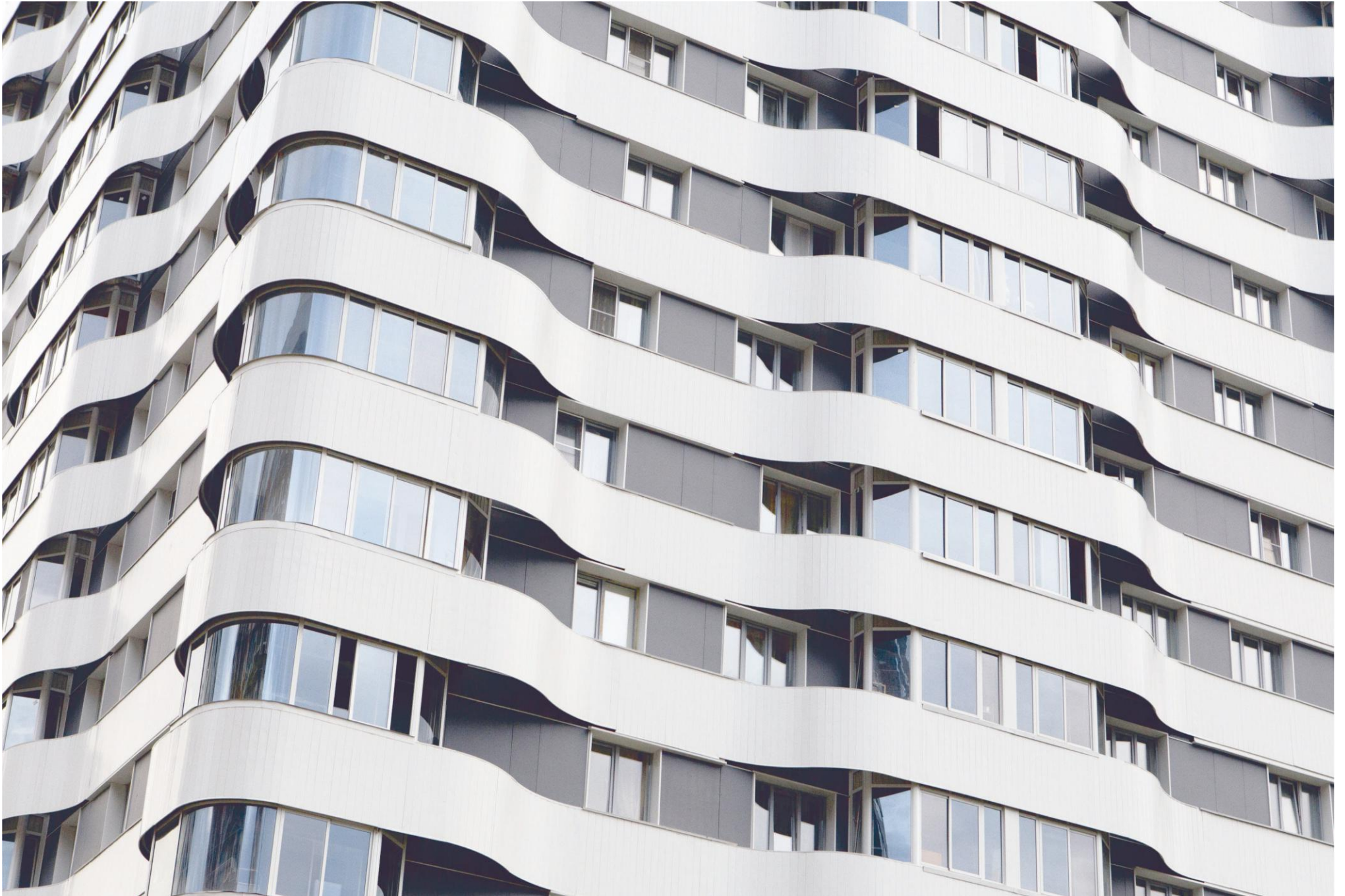
OASIS HOUSING ESTATE, NOVOSIBIRSK
