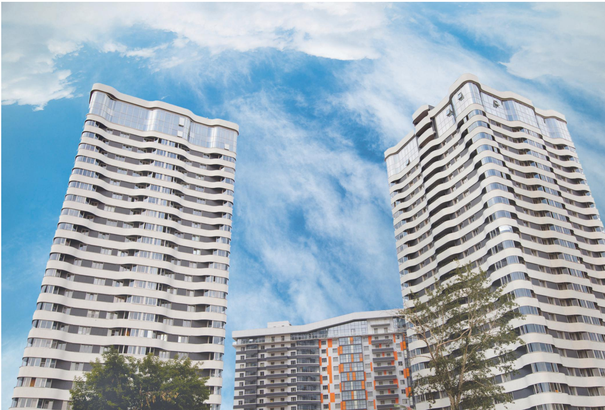
OASIS HOUSING ESTATE, NOVOSIBIRSK
