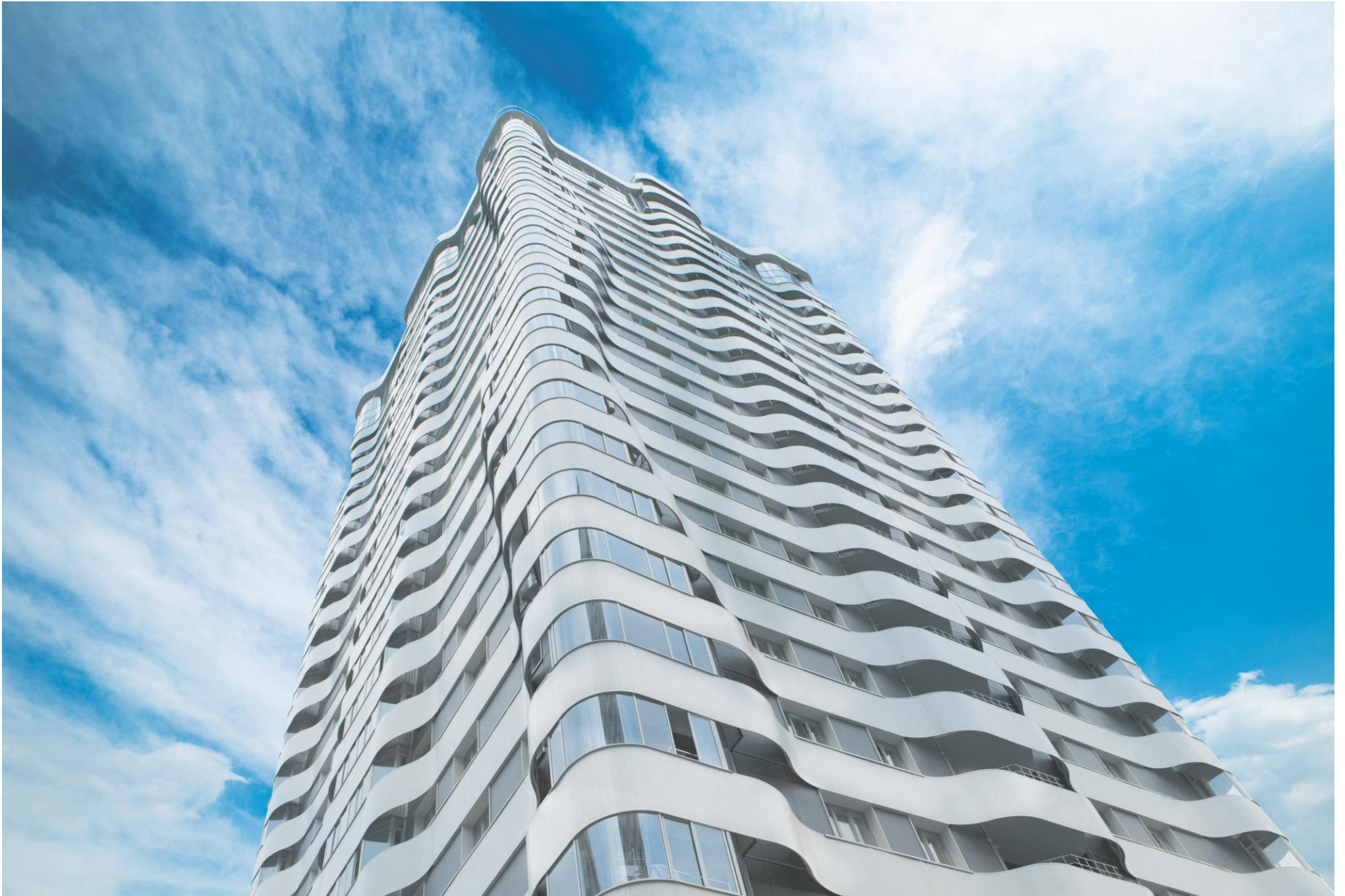
OASIS HOUSING ESTATE, NOVOSIBIRSK
